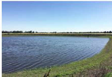
Reservoir dam of Kagome Australia Pty Ltd.
