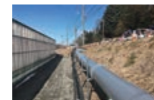
We are using the Fujimi Plant's waste warm water and CO 2 contained in boiler exhaust gas for the cultivation of tomatoes at a nearby farm.
